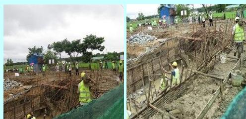
The construction workers provided a measurement to dig the land. The testing concrete is 7days concrete strength gained 65 percentages of trial mix design strength to start work. Consultants confirm to start work the foundation if the testing concrete is 7days concrete strength gained 82 percentages. Currently, 42 workers are working at this site. They dug the total 9 feet for foundation.
