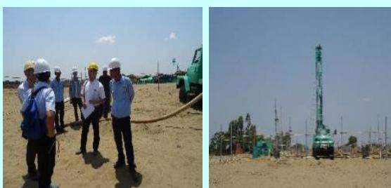
The Water Supply System for the relocation site of zone B has been started since the beginning of April. This Water Supply System includes digging of a deep well with 130m (429 ft), construction of an iron removal plant and an overhead tank. The water from the overhead tank will then distribute water to each household with pipelines. The digging of a deep well has been carried out by a machine. Water Expert from IRP team made supervision to the contractor of this Water Supply System.
