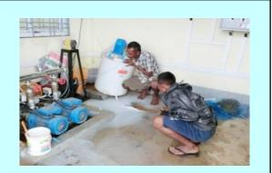
In order to check the water supply system and toilets conditions, TSMC visited to the relocation site on 6<sup>th</sup> and 11<sup>th</sup> June 2018. JET gave the instruction to PAP about the "Chlorine Dosing Operation Procedure" of water supply system. Water sample from the tank will be taken and tasted in every 6 months.
