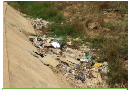
Rubbish at the creek near 6 th Street
