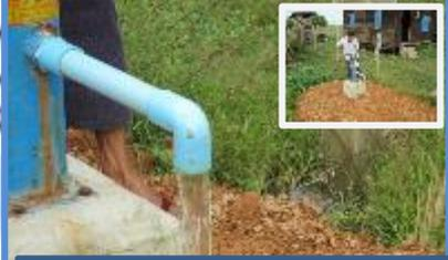
Hand pump is functioned. Water is clean and has no sand, no clay but it has smell of mud. People are using this well for washing.
