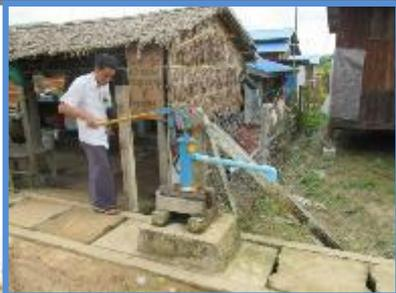
Hand pump isn't functioned very well. The washer needs to be repaired. A lot of water needs to be poured every time before pumping. People are using this well for washing.
