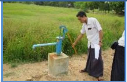
Hand pump is functioned. Water is clean and has no sand, no clay, and no smell. People are using this well for cooking and washing. Sometimes they are drinking.
